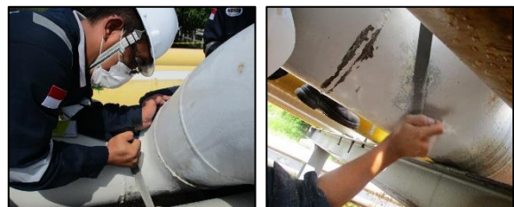
Figure 4. Surface Preparation
