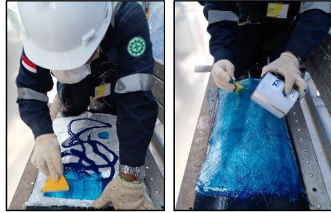
Figure 14. FRP (Composite Wrapping) Preparation
