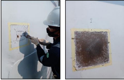
Figure 10. Surface Preparation
