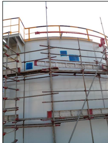
Fig 16. Applied Cold Welding works on all Tank Defects
