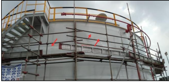
Fig 17. Finish Coating on Cold Welding Works
