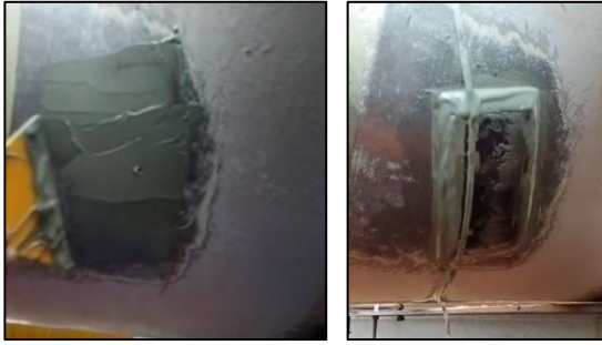
Figure 5. Adhesive and Patching Application
