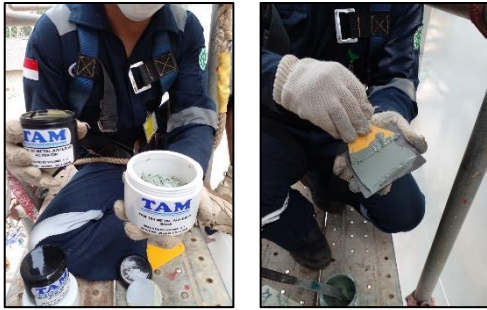
Figure 11. Metal Adhesive and Patching Preparation
