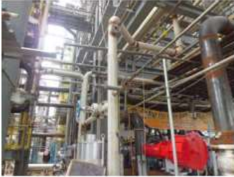
CONDITION ON SITE
