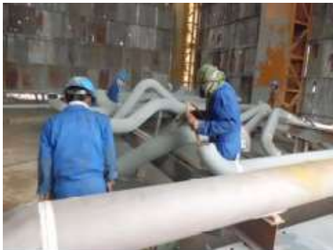
COATING PRIMER APPLICATION
