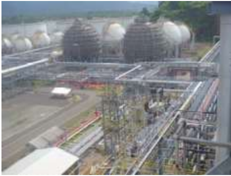
CONDITION ON SITE
