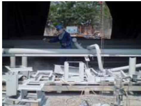
COATING INTERMEDIATE APPLICATION
