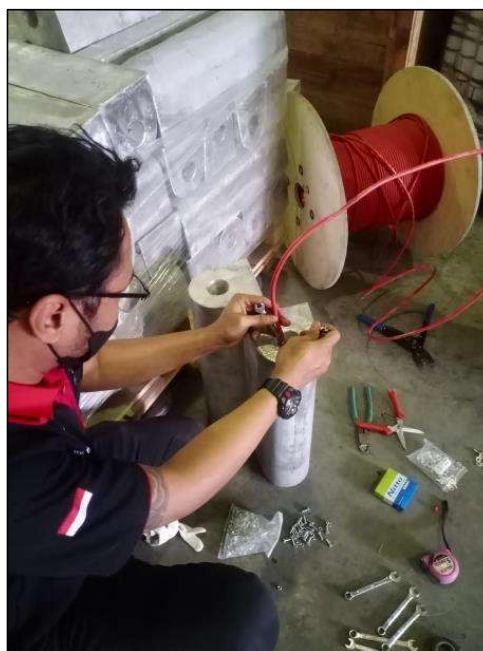
2. Cable Anode Connection
