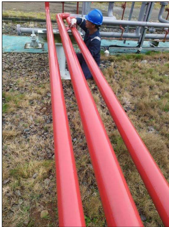
Dokumentasi TAM Pipeline Coating di Pertamina EP Asset 2 Prabumulih - Cat Hydrant Pipeline
