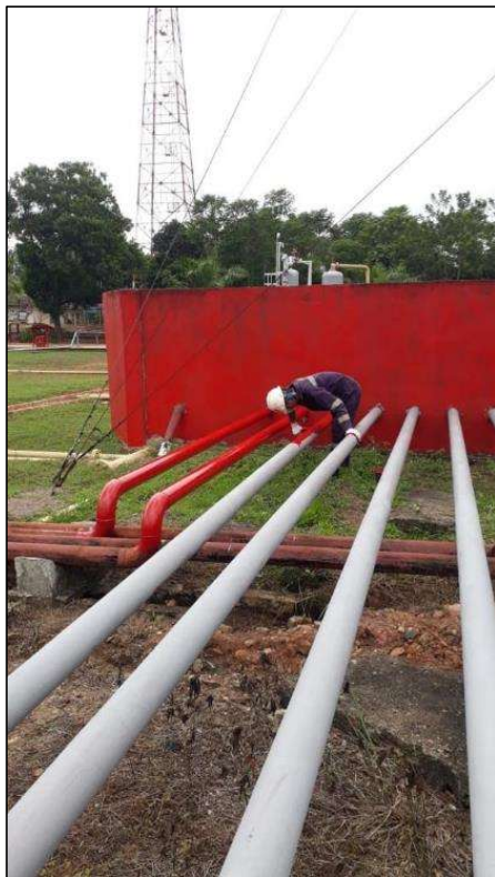
Dokumentasi TAM Pipeline Coating di Pertamina EP Asset 2 Prabumulih - Cat Hydrant Pipeline
