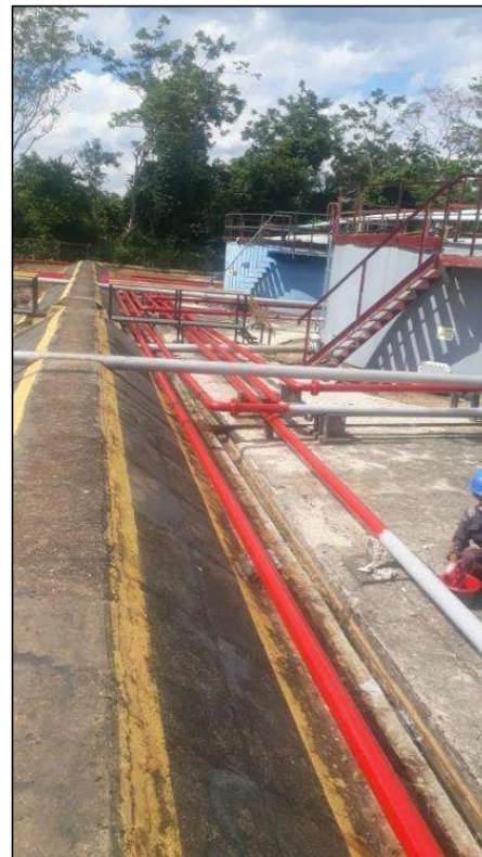
Dokumentasi TAM Pipeline Coating di Pertamina EP Asset 2 Prabumulih - Cat Hydrant Pipeline
